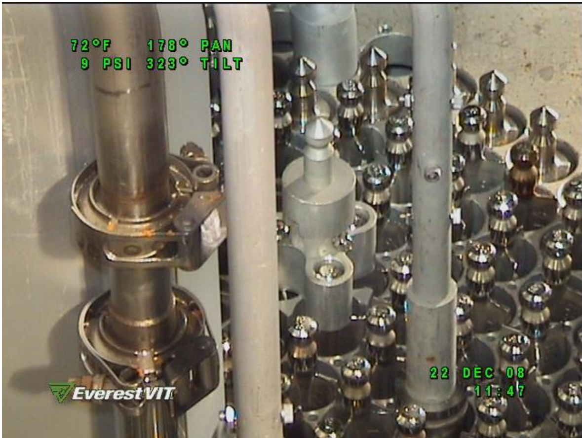
Figure 19. Photograph, Tri-Element Facility
